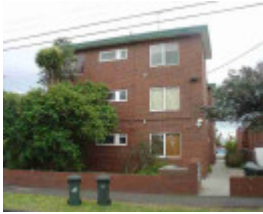
fitzroy north holden street fitzroy north holden street 125
