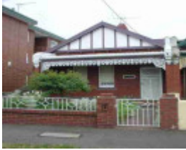
fitzroy north holden street fitzroy north holden street 127
