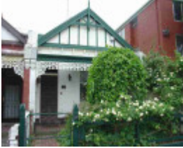
fitzroy north holden street fitzroy north holden street 133
