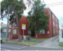
fitzroy north holden street fitzroy north holden street 137
