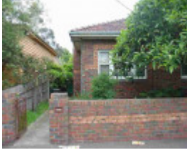
fitzroy north holden street fitzroy north holden street 147
