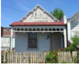
fitzroy north holden street fitzroy north holden street 150
