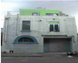
fitzroy north egremont street fitzroy north egremont street 35
