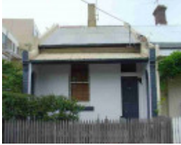
fitzroy north napier street fitzroy north napier street 499
