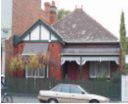
fitzroy north nicholson street fitzroy north nicholson street 496
