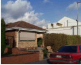
Fitzroy North Pilkington Street 2.JPG
