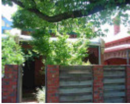
fitzroy north holden street fitzroy north holden street 209
