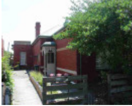
fitzroy north holden street fitzroy north holden street 215
