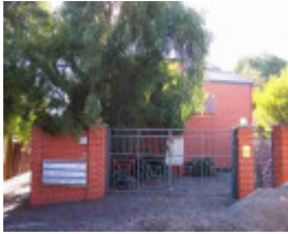
fitzroy north mckean street fitzroy north mckean street 221 unit 10
