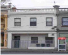
fitzroy north nicholson street fitzroy north nicholson street 448
