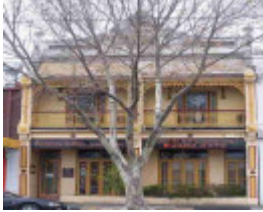
fitzroy north nicholson street fitzroy north nicholson street 452
