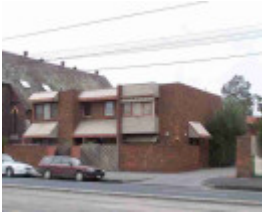
fitzroy north nicholson street fitzroy north nicholson street 466 unit 1-22
