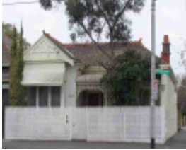
fitzroy north nicholson street fitzroy north nicholson street 492
