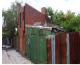
Dairy - Rear of 242 Scotchmer Street.JPG
