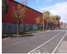
Former Coal Shed.JPG
