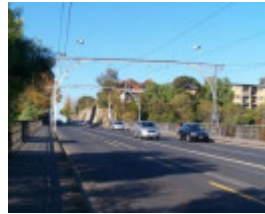
Victoria Street Bridge
