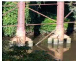
Victoria Street Bridge
