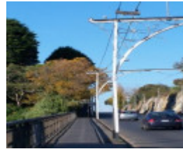
Victoria Street Bridge
