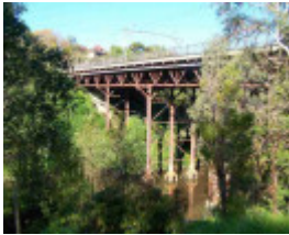
Victoria Street Bridge
