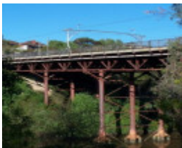
Victoria Street Bridge
