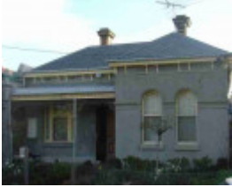
fitzroy north rushall crescent fitzroy north rushall crescent 73
