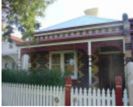
fitzroy north rushall crescent fitzroy north rushall crescent 85
