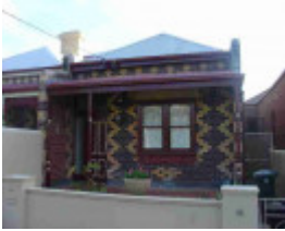
fitzroy north rushall crescent fitzroy north rushall crescent 87
