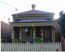
fitzroy north rushall crescent fitzroy north rushall crescent 89
