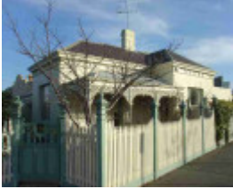
fitzroy north rushall crescent fitzroy north rushall crescent 97
