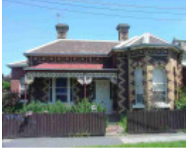
fitzroy north rushall crescent fitzroy north rushall crescent 103
