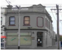
fitzroy north nicholson street fitzroy north nicholson street 446
