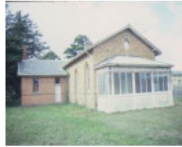
1 smythesdale court house front view jun1984
