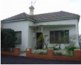
fitzroy north park street fitzroy north park street 222
