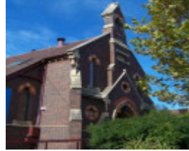
Former Methodist Church
