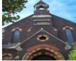
Former Methodist Church
