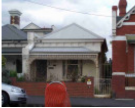
Fitzroy North Rae Street 366.JPG
