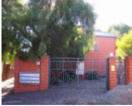
fitzroy north mckean street fitzroy north mckean street 221 unit 8
