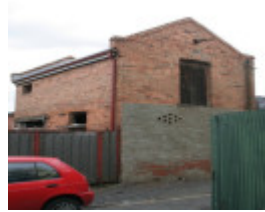
Rear of 118 Michael Street
