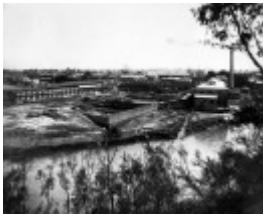
1918 - Yarra Falls construction.jpg
