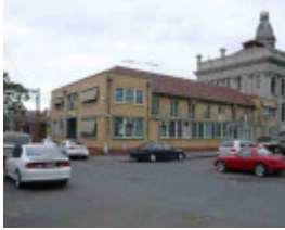
Fitzroy Police Station
