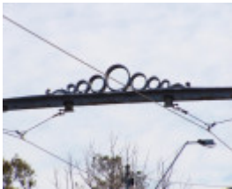
Tram poles - Swan Street
