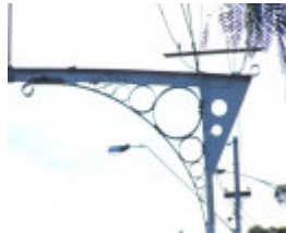
Tram poles - Swan Street
