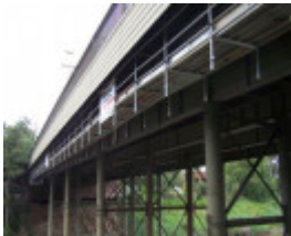
Yarra River Bridge
