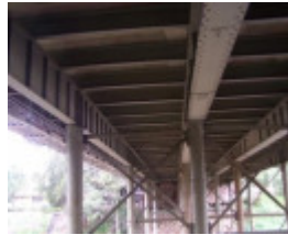
Yarra River Bridge
