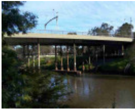
Yarra River Bridge
