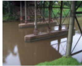
Yarra River Bridge
