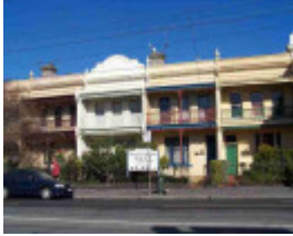
Byrne's Arcade Terrace - 320 Victoria Street
