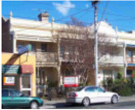
Byrne's Arcade Terrace - 324 Victoria Street
