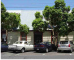
Richmond Orderly Room - 26 Gipps Street
