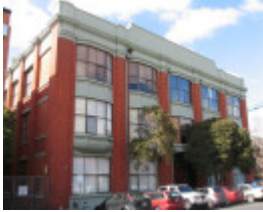
120 Cambridge Street - West Elevation from Cambridge Street
