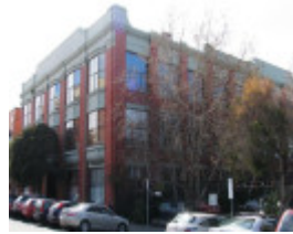
120 Cambridge Street - West Elevation from Cambridge Street
