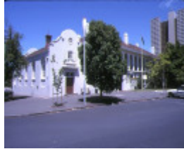
1 south melbourne court house & police station bank street south melbourne front view
