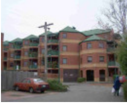
fitzroy north st georges court fitzroy north st georges court 3 unit 1-41
