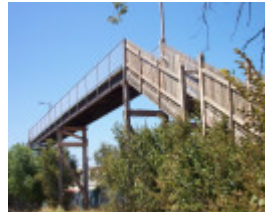
Former Footbridge near Napier Street
