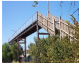
Former Footbridge near Napier Street
