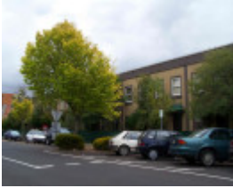
Fitzroy North Miller Street 9-19.JPG
