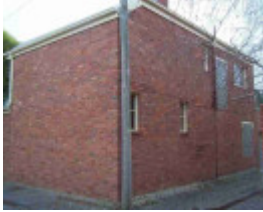
fitzroy north rowe street fitzroy north rowe street 66 unit 2
