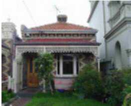
fitzroy north rushall crescent fitzroy north rushall crescent 37
