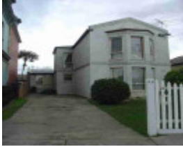
fitzroy north rushall crescent fitzroy north rushall crescent 43
