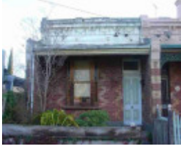
fitzroy north rushall crescent fitzroy north rushall crescent 59
