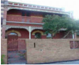
fitzroy north rushall crescent fitzroy north rushall crescent 65
