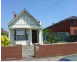
fitzroy north rushall crescent fitzroy north rushall crescent 113
